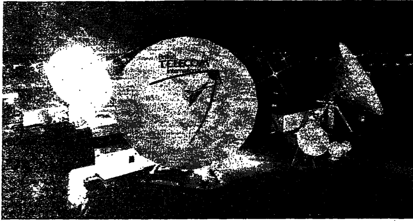
This is Teleport in London's dockland, the first international earth station to be installed in a city. It transmits six television channels to cable TV networks in the UK and Europe from three 43ft diameter aerials
